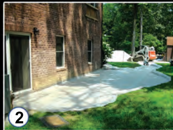
Install Geotextile Fabric
