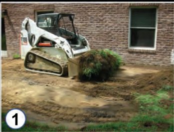
Excavate Job Site
